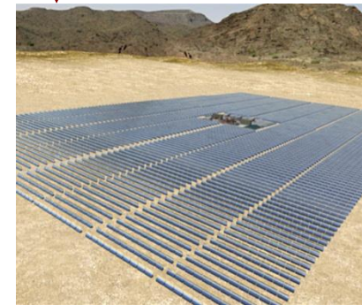
Solana CSP power plant. 280 MW. AZ, USA
